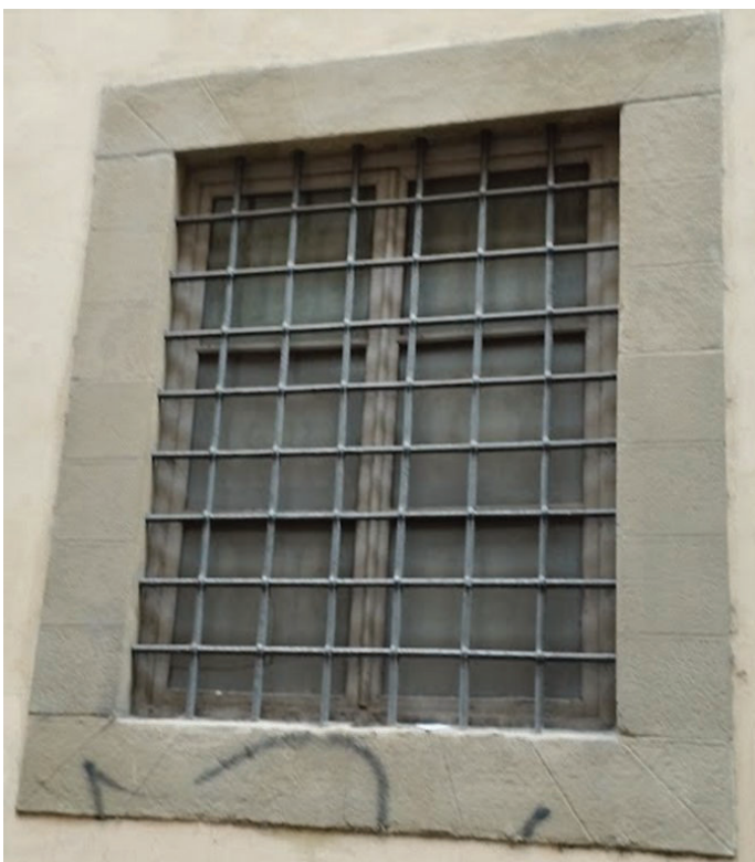
Figure 3: Grate made of pierced vertical rods and plain horizontal non-pierced rods passed through the pierced holes rods (Photo: M. Bram).
