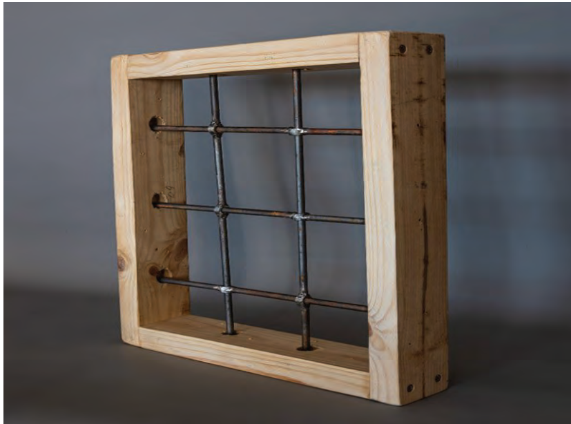
Figure 2. Mock-up of iron grate installed in a opening (Photo: A. Pintel).
