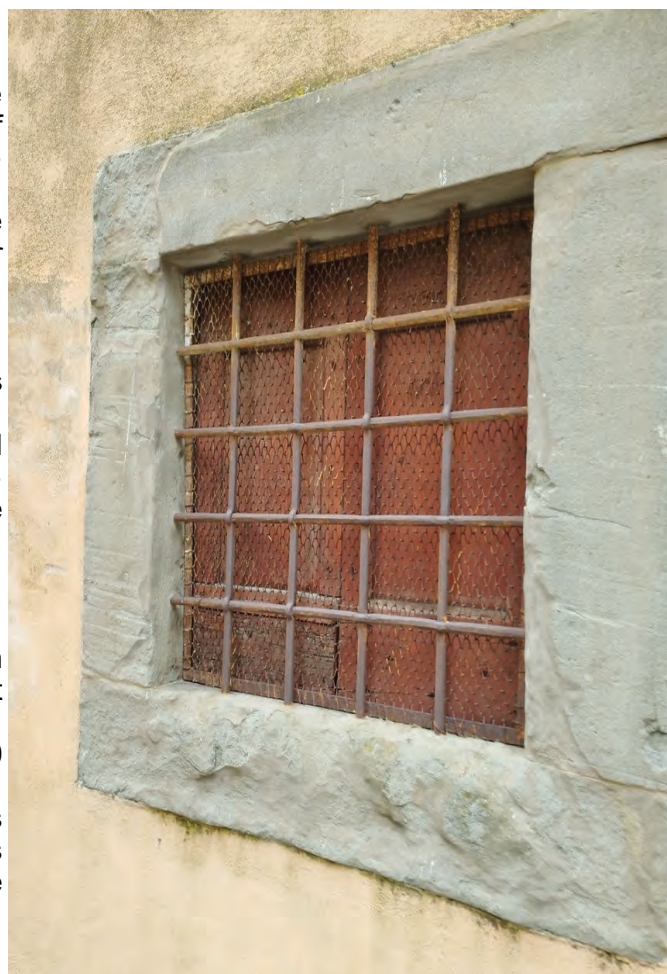
Figure 1. Alternative-penetration-rod iron grate, Florence, Italy (Photo M. Bram).
